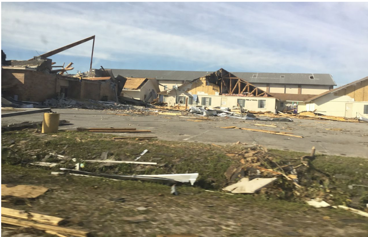
Hurricane Michael damages the local infrastructure, including this church in Callaway. (Photo is public domain.) (National Oceanic and Atmospheric Administration.)
